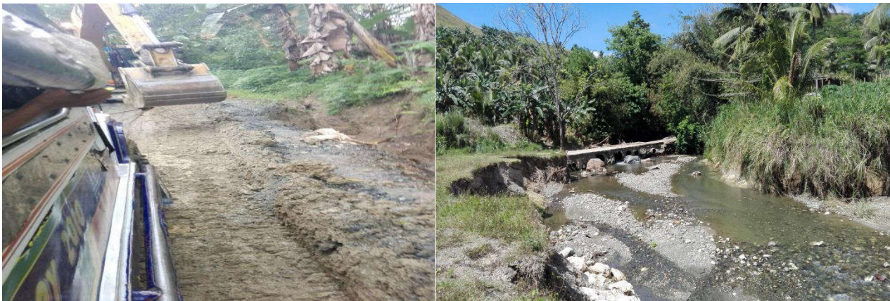
Photo 5: Road going to Tumpagon. Photo 6: Road going to Nangaon
